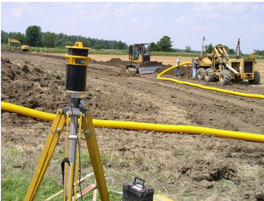
Figure 8. Installing drain tile in agriculture fields to aid in lowering water table. (Huntington Township).
