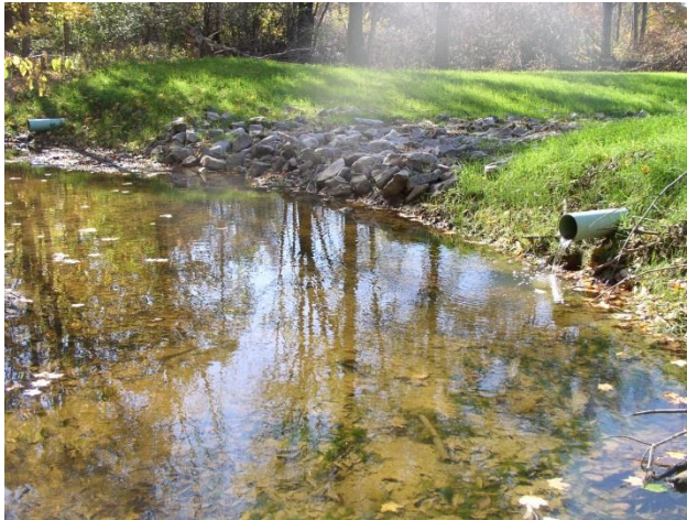
Figure 5. Swales and drainage tile flowing into a natural stream is often the best outlet for storm water.
