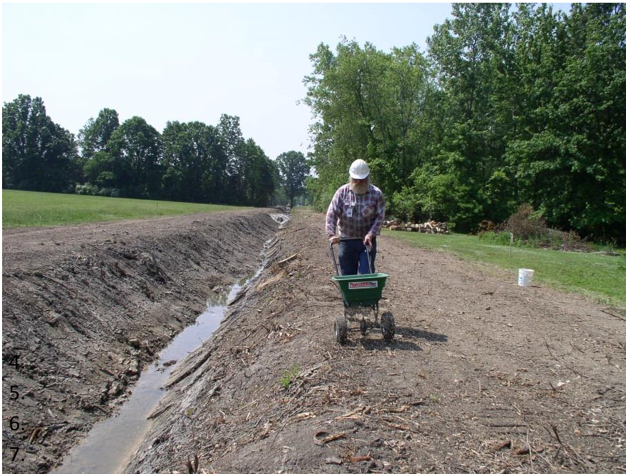
Figure 7. Newly constructed and seeded ditches, completed through ORC, will aid in storm water flow and improve property value (Elyria Township).
