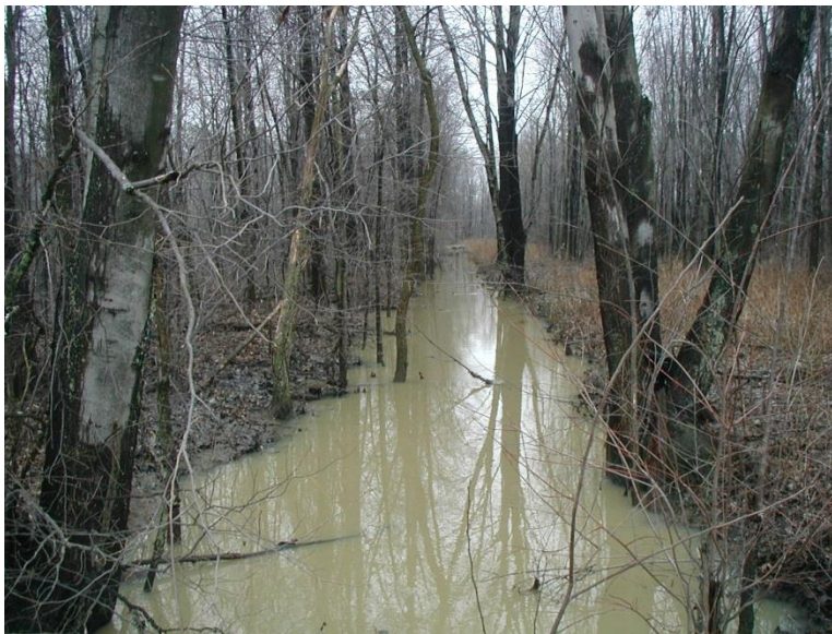
Figure 6. Ditches filled with trees, brush, sediment and other debris have limited capacity and require periodic maintenance (New Russia Township).
