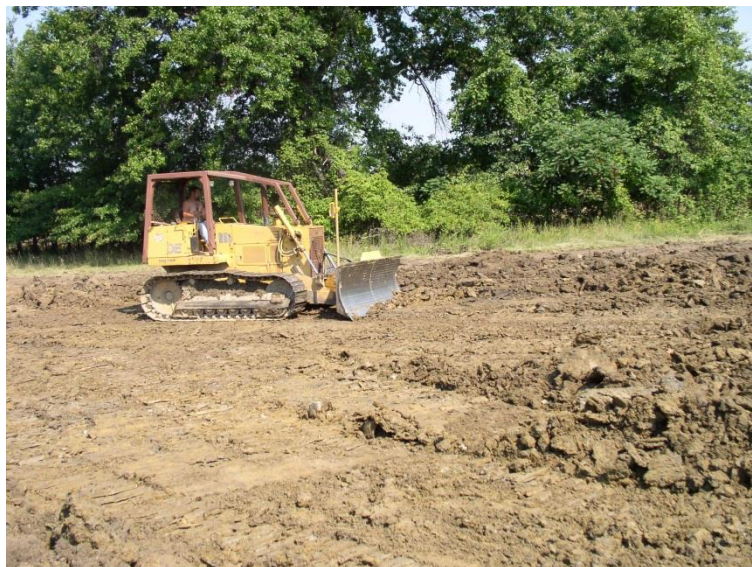
Figure 3. Excavated soil material placed in the wrong area can cause disruption of drainage patterns that results in flooding and standing water.
